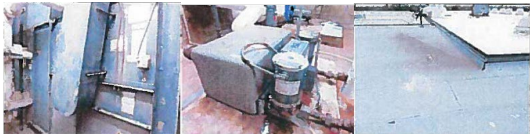
Extremely old HVAC air handling units and condensing return pump; Older roofing installation with multiple soft spots and water ponding throughout
